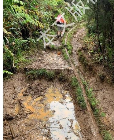
The lateral inclination of the walking surface (3 to 5%) is provided for this purpose. A lateral downstream inclination is the most frequent. A lateral upstream inclination is a good idea if there is a risk of users slipping into a ravine, but it requires longitudinal drainage and transverse drainage pipes.
