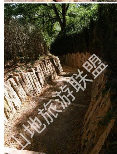
If the work is deep, it is recommended to first clear the upper humus (the layer rich in organic matter) and not to mix it and pile it up with the basement materials. After building up the walking area of the trail, it will be advisable to spread this humus on the surface to allow faster re-vegetation.
