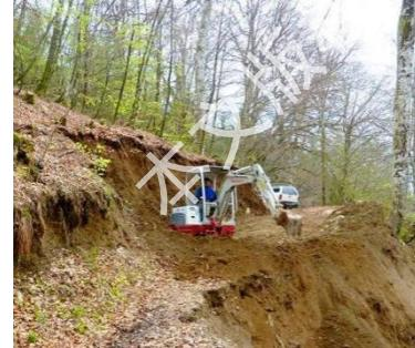
Excavation work to pass a trail on a slope is often accompanied by the construction of retaining walls. These are installed downstream to strengthen the foundation of the trail or upstream to prevent the collapse of the dug embankment.
