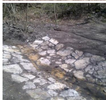
The greater the longitudinal slopes of the trail are, and the more frequent heavy rainfall is, the shorter the distances between each water bar must be (varying between 5 m and 60 m). Their cleaning is part of the routine maintenance work.
